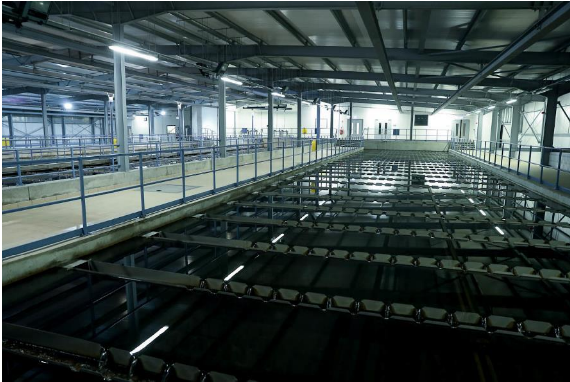
Leixlip Water Treatment Plant, County Dublin
