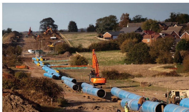
Pipeline corridor showing pipe before trenching and welding
