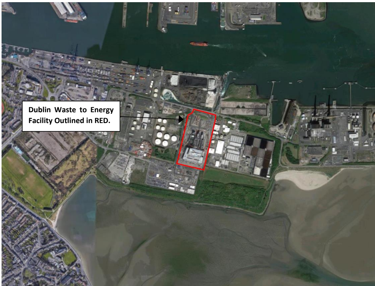
Figure 3.4: Dublin Waste to Energy Facility
