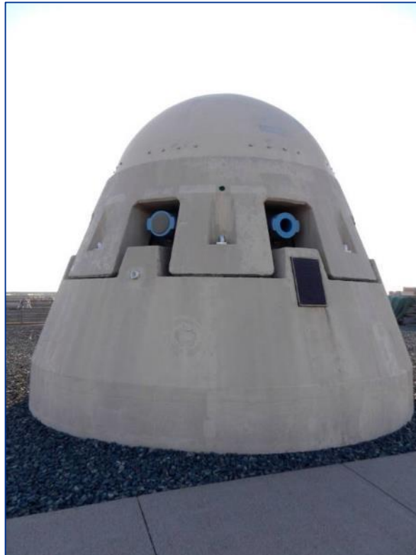
Figure 43: Typical Precast Concrete Protection for Outfall Riser
