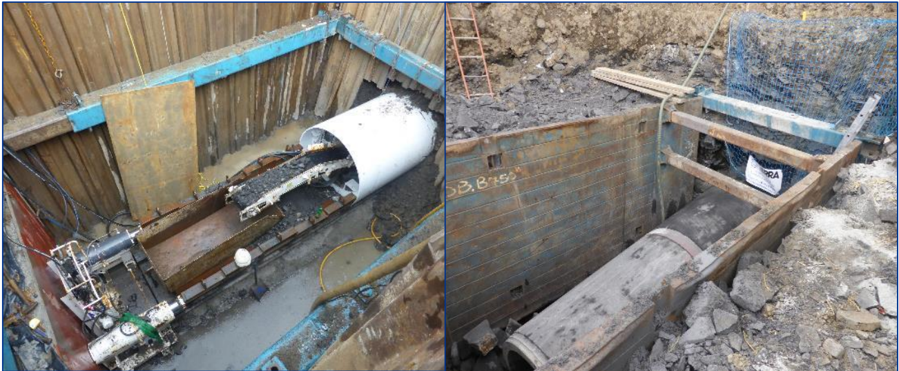
Figure 16: Tunnel Jacking Launch Shaft
