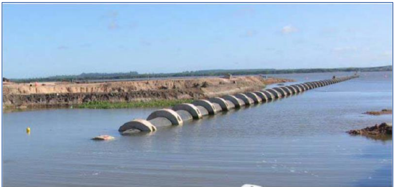
Figure 38: Step 4 - Submersion by water filling/air evacuation - copyright PipeLife Norge AS
