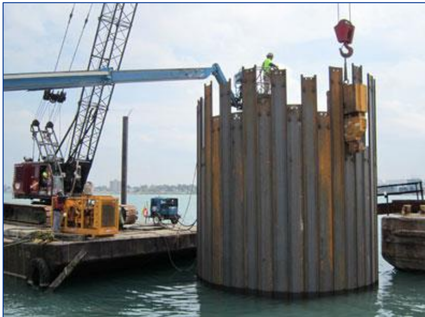
Figure 28: Construction of Cofferdam
