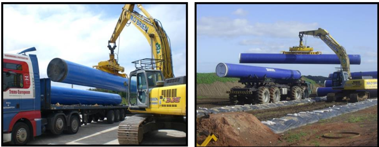
Figure 12: Pipe Lengths being unloaded using a Vacuum Lift
