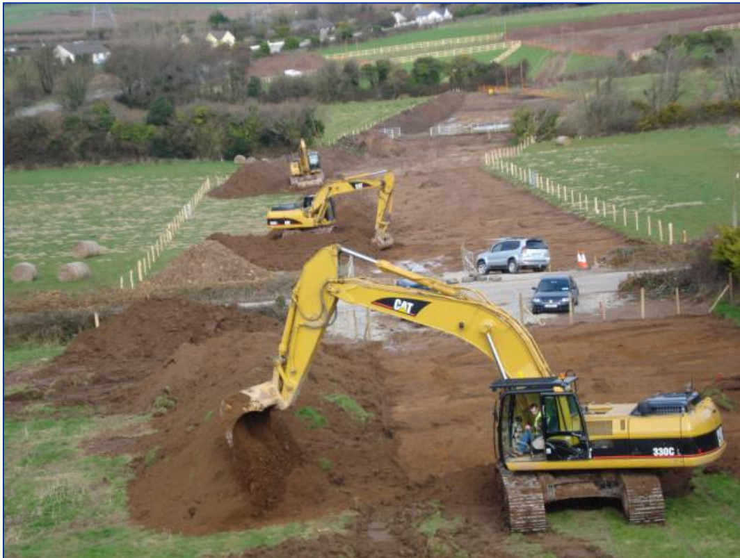
Figure 11: Typical Construction Corridor – Topsoil stripping
