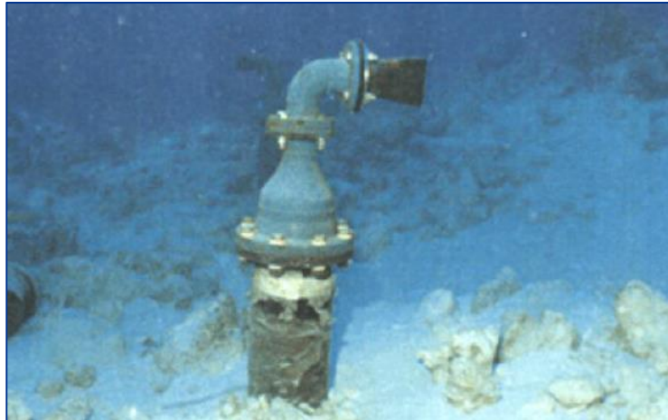
Figure 42: Marine Riser above Seabed
