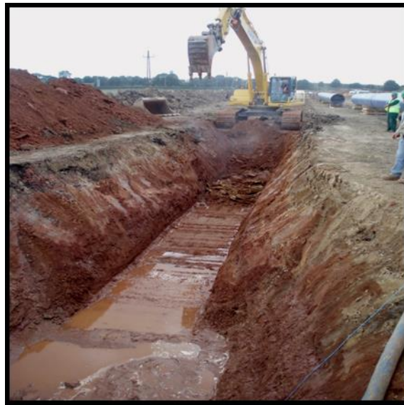
Figure 14: Trenching using Excavators
