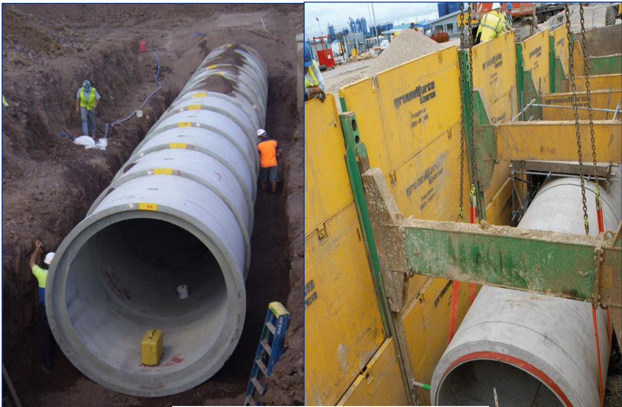
Figure 15: Open Cut Method for Sewer Construction
