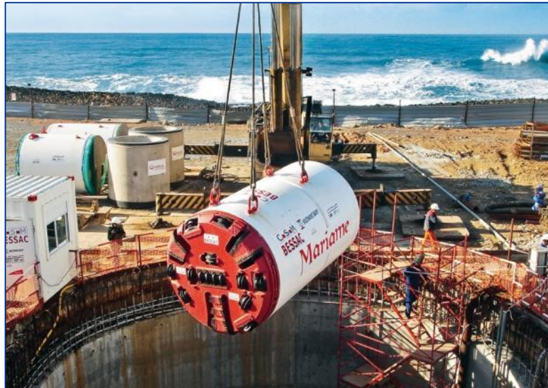
Figure 24: Micro-Tunnelling Machine lowered into Tunnel Shaft
