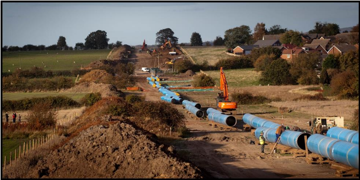
Figure 13: Pipe Stringing along the Pipeline Corridor
