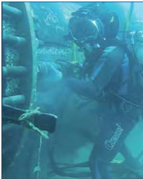
Figure 39: Subsea flanged connection between sections by divers
