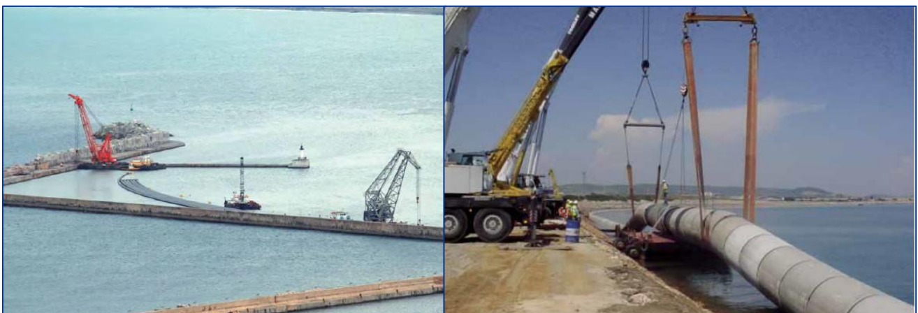
Figure 35: Typical Ballasting and Pipe Assembly Location off Quay wall
