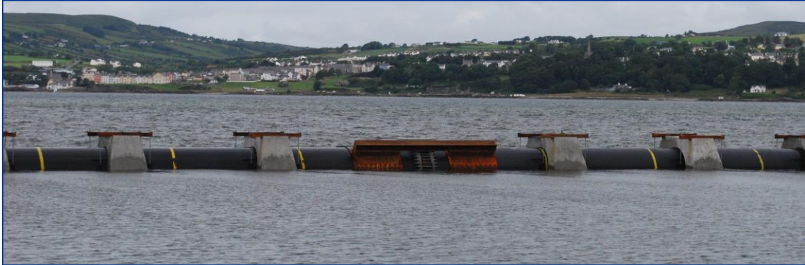
Figure 34: Connection of Long Pipe Strings
