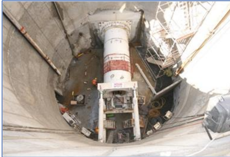
Figure 25: Micro-Tunnelling Machine Launch Shaft
