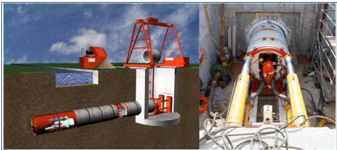
Figure 27: Tunnel Schematic & Micro-Tunnelling Machine commencing
