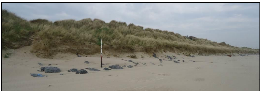
Plate 3: View looking North at foot of sand dunes, at a point where the access route will turn eastwards across the beach. The dark grey boulders reflect the line of rock-armour protection inserted to prevent coastal retreat.
