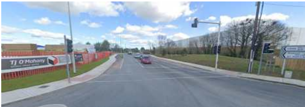
Figure 13b: Photo of Current L3125 arm on Kilshane Cross (Signalised) Junction (Source: Google Maps)
