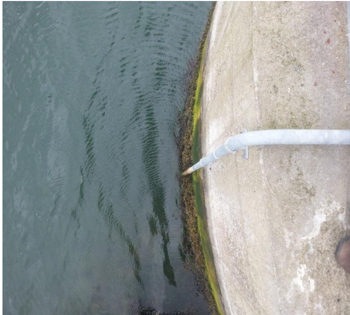
Figure 14. Marine Institute Bubble Tide gauge. TechWorks fastened a pole and Pressure tide gauge to the base of this pipe.
