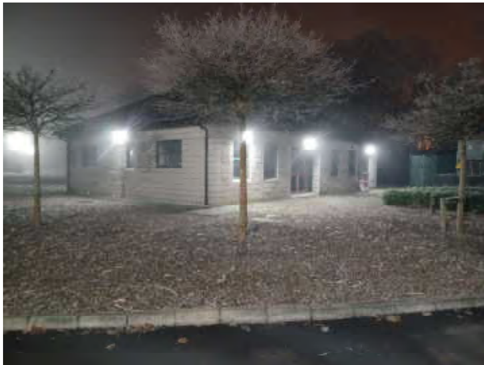
Figure 11-17: Existing Lighting on Buildings
