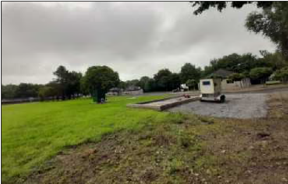
Figure 11-3: WwTP infrastructure classified as buildings and artificial surfaces (BL3) and associated hard stand areas of (BL3)/spoil and bare ground (ED2)/recolonising bare ground (ED3). Grassland classified as amenity grassland (GA2).
