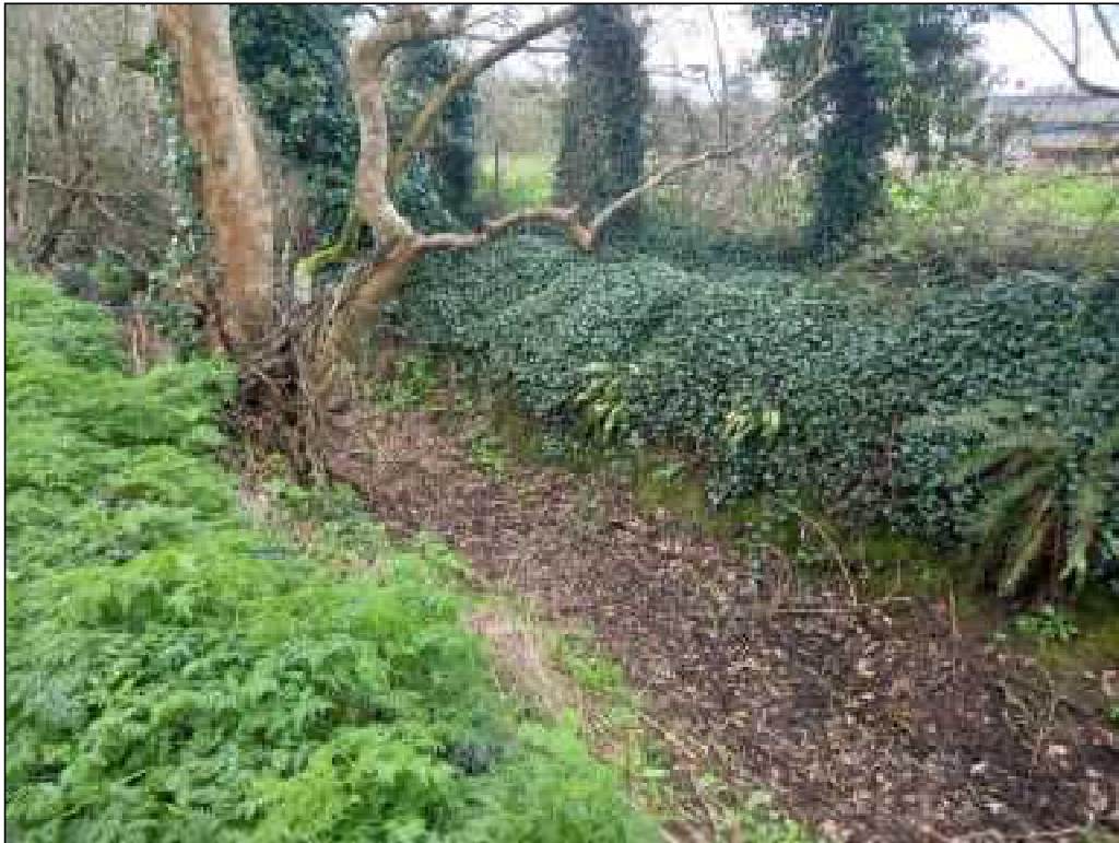
Figure 11-5: Drainage ditch (FW4), dry at the time of the surveys, outside of the eastern boundary.
