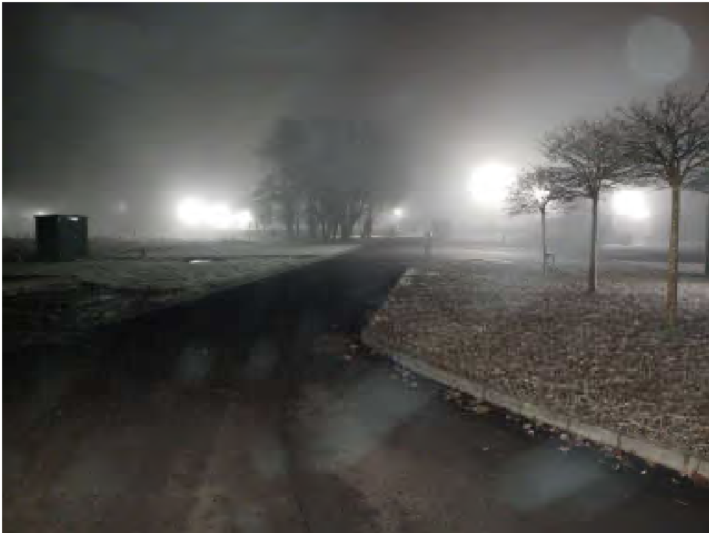
Figure 11-12: Current lighting situation at Castletroy WwTP
