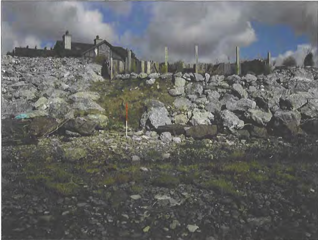
Plate 11: North-facing view of upper foreshore c.550m along pipeline route (see Figure 6 for location); 1m scale.
