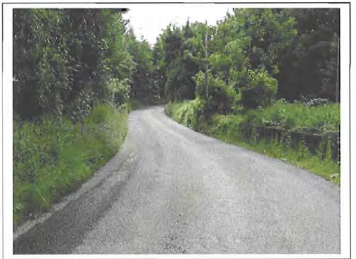
Plate 3.14. Pipeline route along roadway within ZAP of CH8, from northeast
