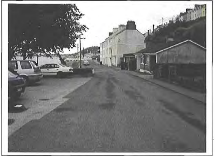
Plate 3.30. Pipeline along roadway at east side of Cobh, from east
