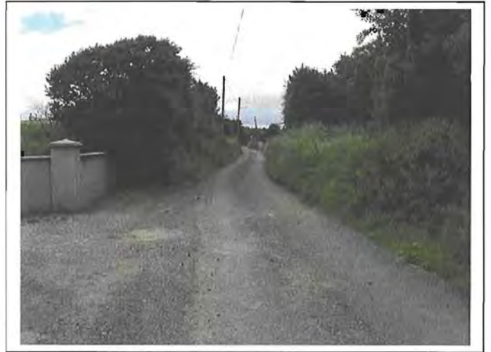
Plate 3.25. Pipe route along roadway in Loughbeg, from east
