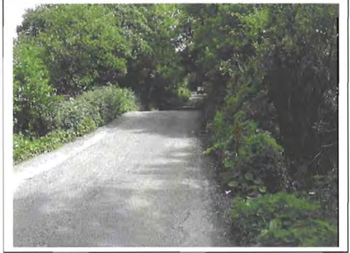
Plate 3.12. View southward over 'Dandy bridge' in Kilnagarry
