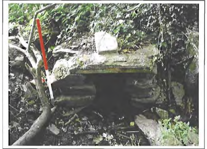
Plate 3.36. CH2, from east
