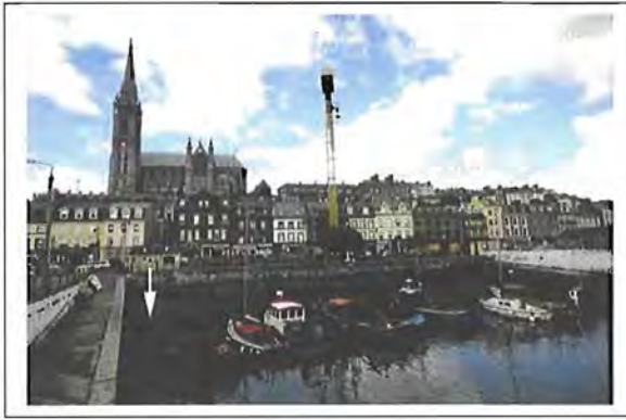
Plate 3.46. Location of major pumping station at West Beach Cobh, from south
