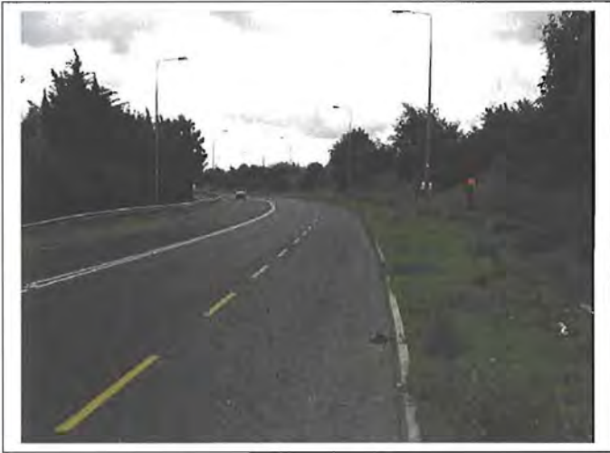
Plate 3.24. Pipe route along N28, from northwest
