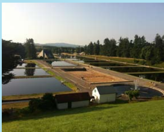
Vartry Water Treatment Plant. Photo: Nicholas O'Dwyer.
