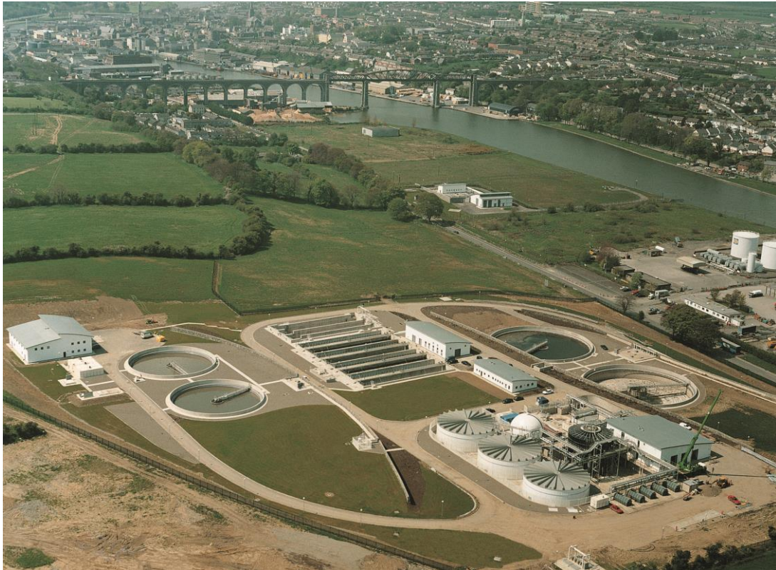
Figure 9.2 – Drogheda Wastewater Treatment Plant
