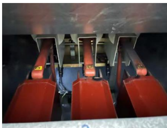
Picture 2: Suspected location of Arc
