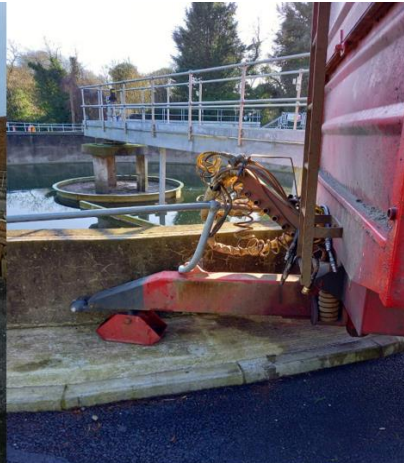
Fig. 2: Sludge trailer collided with clarifier
