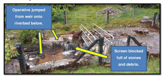
Incident 2: Due to sedimentation build up, an operative was required to rod a pipeline to clear sediment from the RBC outfall. This pipeline was situated 5m into a river. This task/activity occurred several times a year. There was no safe access/egress provided to carry out this task/activity safely.
