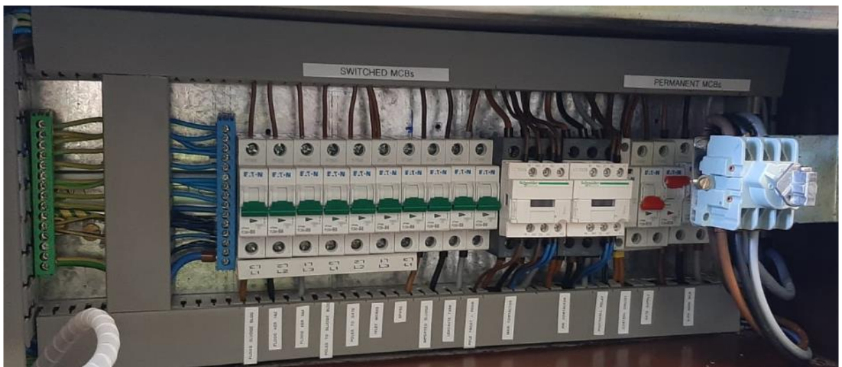
Picture 3: Finished panel, all MCBs labelled & drawings updated.
