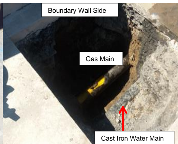
Fig 3 Excavation 2 Services Layout
