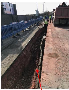
Partial trench collapse during water saddle valve repair works.
