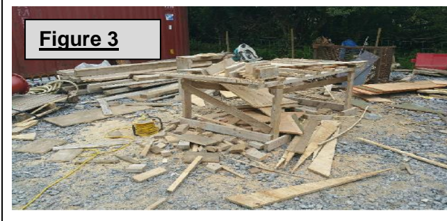
Figures 1-3 above were taken during IW HSQE Inspections on Irish Water sites and demonstrate examples of poor housekeeping practices.
