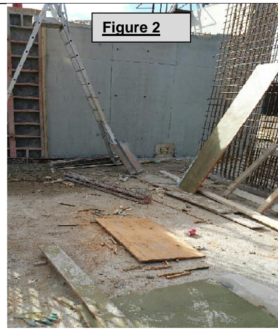
Figures 1-3 above were taken during IW HSQE Inspections on Irish Water sites and demonstrate examples of poor housekeeping practices.
