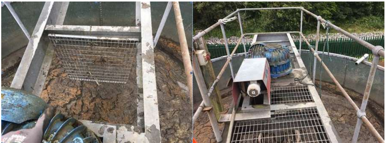
Photo 1: Incident scene where High Potential Near Miss occurred.
