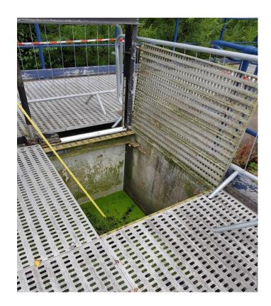
**Photo 1: Grid flooring over Inlet Works**
