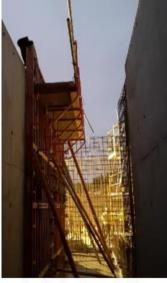
No handrail at the end of the working platform.
