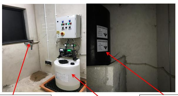
Redundant fill pipe from disused hydrofluorosilicic acid bulk storage tank (located at the opposite side of wall)
